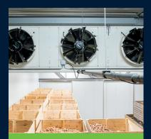
Equans' solution A sustainable condensation drying system that produces both hot as cold air: without gas heaters and with a lower  $CO_2$ -footprint.
